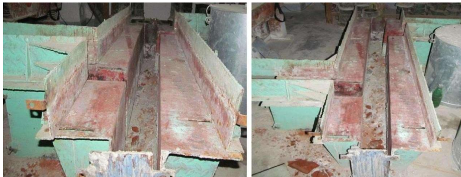
The steel frame used to cast RC T-beams
