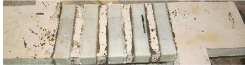
T-shaped beam strengthened using completely wrapped GFRP beams.
