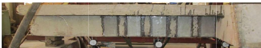
T-beam Strengthened with GFRP of U-Wrap
